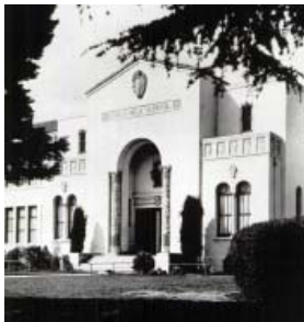
MVHS on Castro Street
